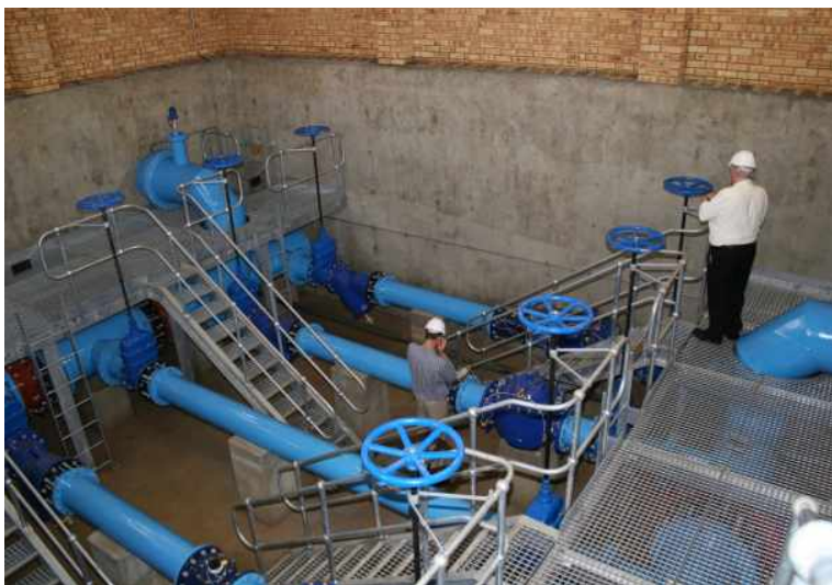
Figure 3: Tim Waldron inspecting one of world's largest Pressure Management installations near Johannesburg
