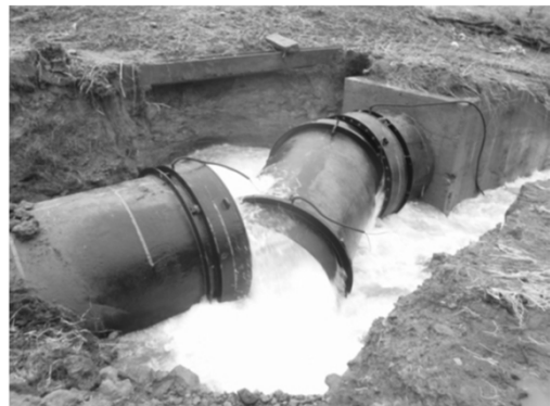
φ2400mm Pipe (Flexible Joint), Sennan-Senen Regional Waterworks by Miyagi Prefectural Government
