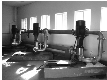
Refurbishment of Perold Booster Pump Station
