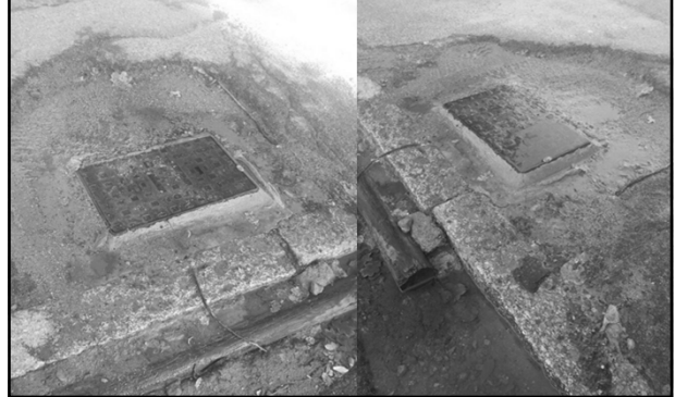
Leak Detection /Repair
