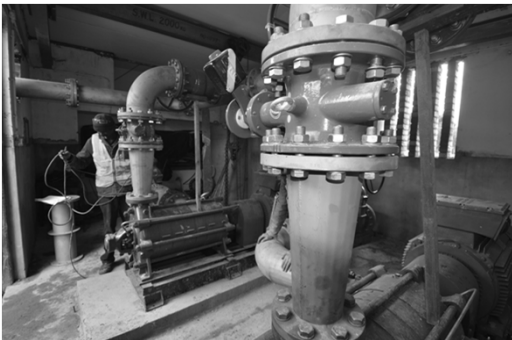
Refurbishment of Ysterbrug Pump Station - 22 August 2013
