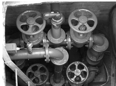
Refurbishment of L`Ideal Close Booster Pump Station - Valve Chamber
